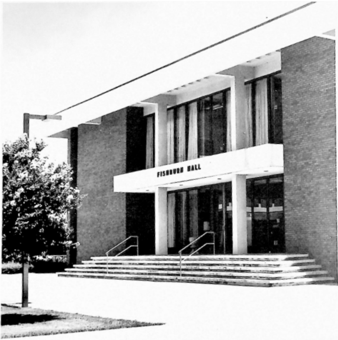
FISHBURN HALL ADMINISTRATION BUILDING
