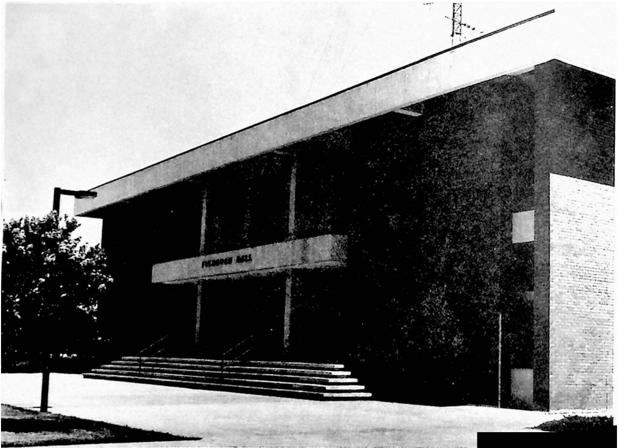
FISHBURN HALL ADMINISTRATION BUILDING
