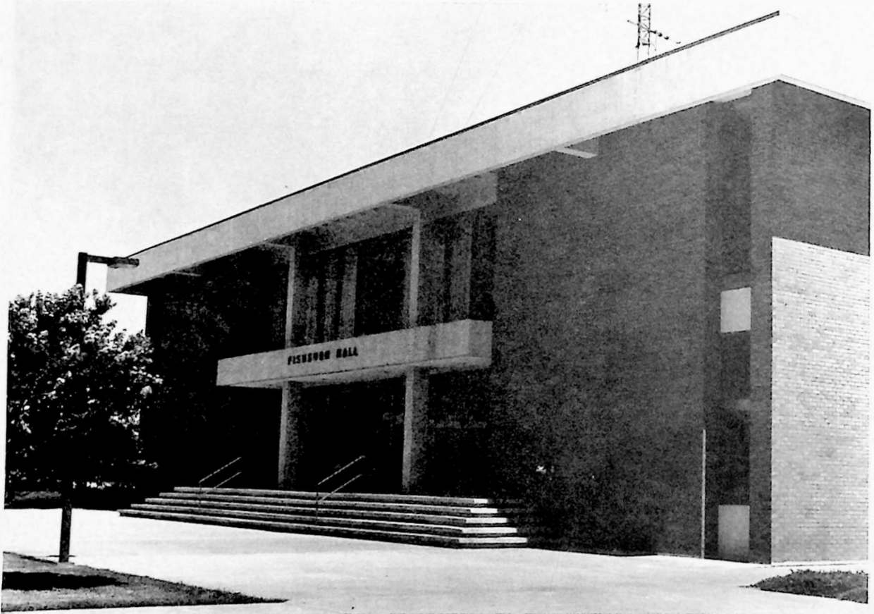
FISHBURN HALL ADMINISTRATION BUILDING
