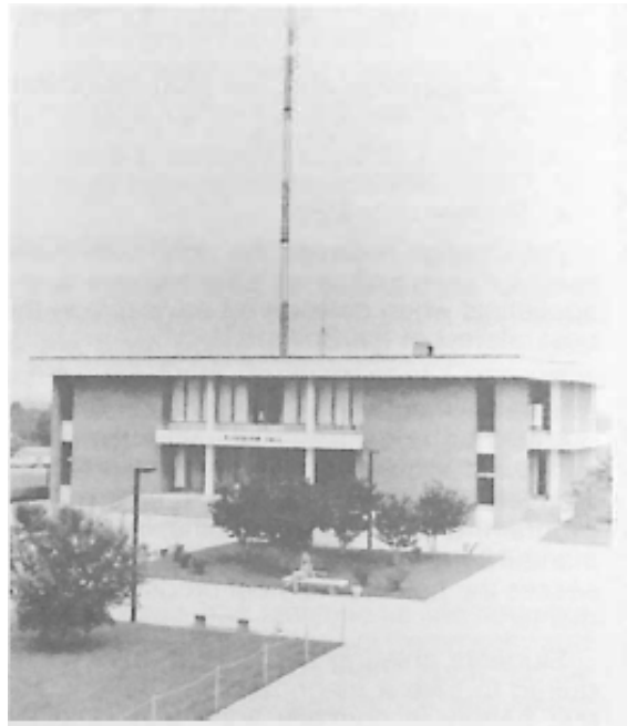
FISHBURN HALL ADMINISTRATION BUILDING
